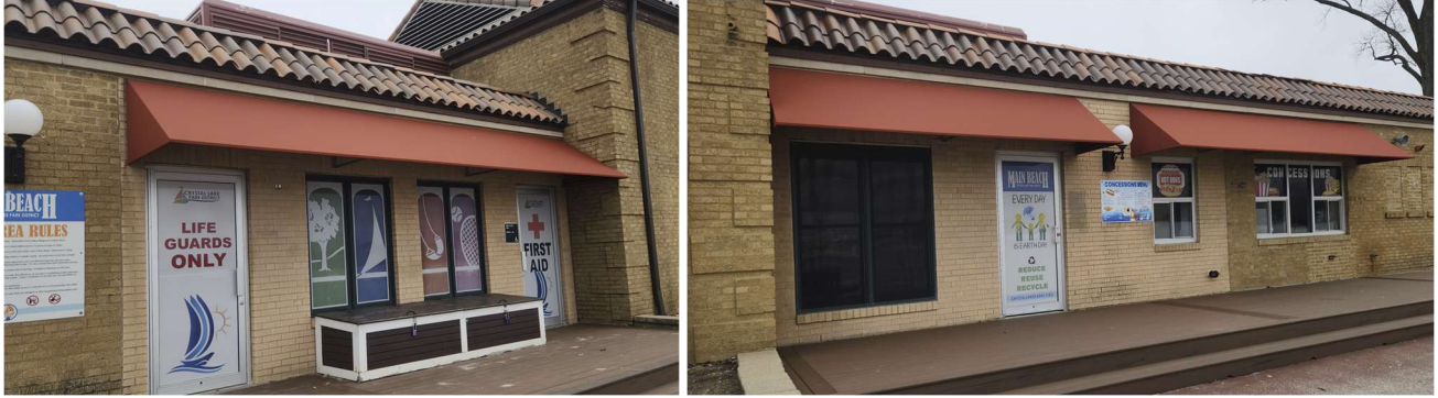
New Fabric on West Awnings
