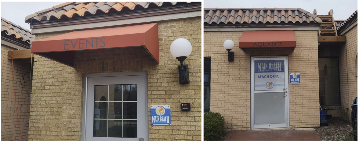
New Awnings over Entrances
