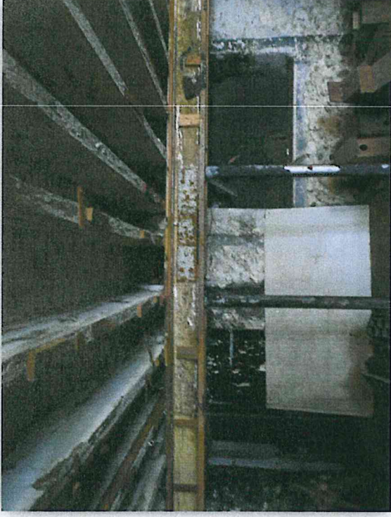
Figure 22 – Structure Supporting Mow Floor
