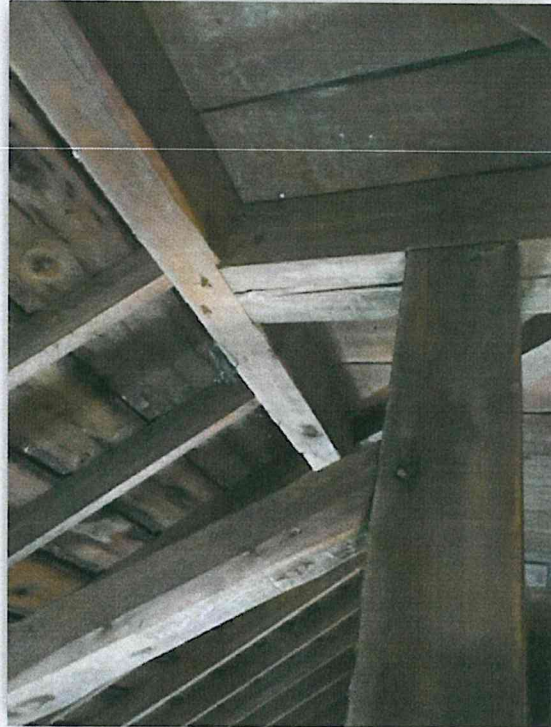
Figure 14 – Side Wall Post with Wall Ties Mortised
