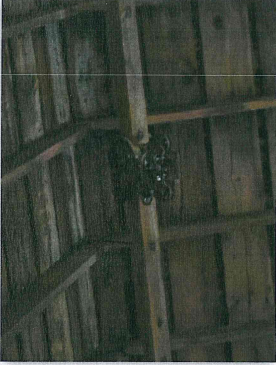
Figure 18 – Hay Fork Trolley on Wood Rail Beam
