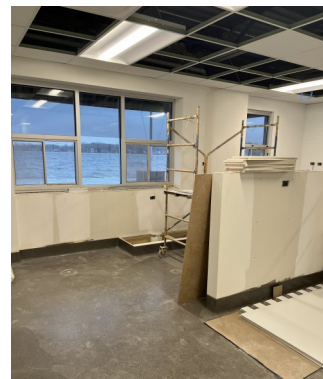
Newly Configured Concessions Prep Area
